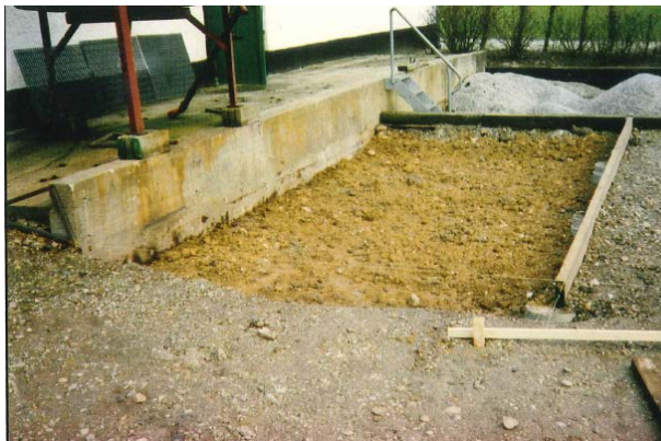
Figure 4. A 60 cm deep pit is excavated and 10 cm of dense clay is placed on the bottom.
