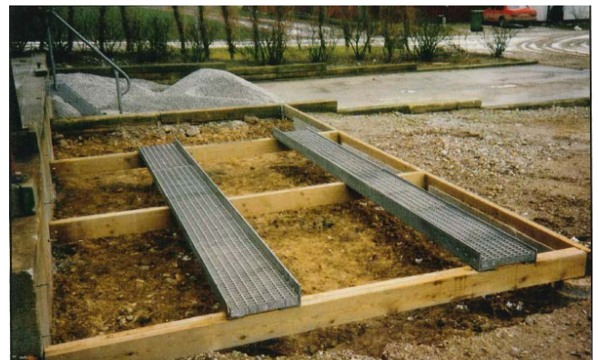
Figure 5. A mesh grid is positioned on top, so that the biobed can be used for parking, washing and filling the sprayer, to avoid point-source pollution from any accidental spillage.
